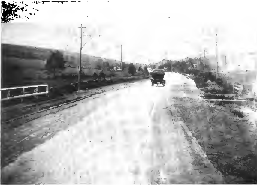
STATE HIGHWAY AT SPENCER, MASS., PAVED WITH HASSAM CONCRETE.
